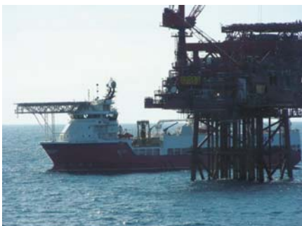
Fig. 3. Source vessel operations near installations.
